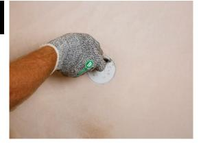
Remove the central area with a sharp hooked blade knife (or hole saw), being careful to avoid any wires within.
