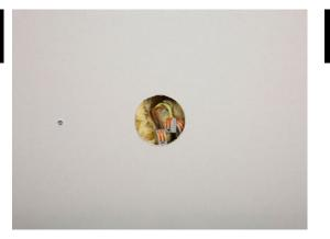
Push wires centrally into recess and staple BeadMaster cover plate in place.
