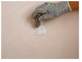
Locate and tap lightly with the head of a screwdriver (or similar) on central area which will loosen the plaster on the face of the bead. Continue until the cut line is visible.
