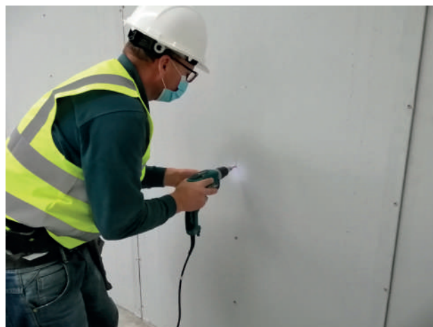
Fixing of SECOLITE® Cement Board with SECOLITE® Screws
