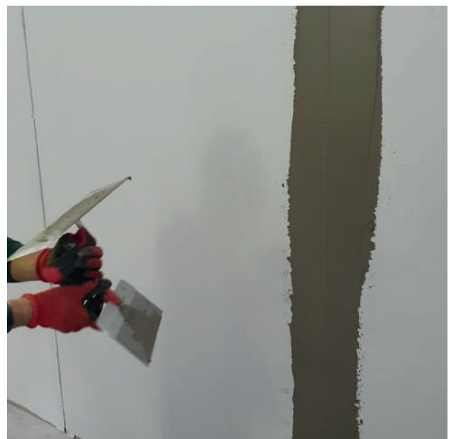
Covering SECOLITE® Joint Tape with SECOLITE® Joint Filler
