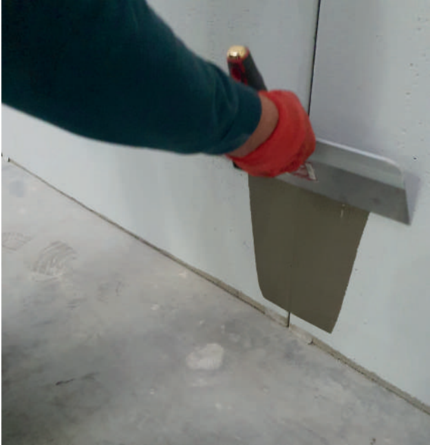
Applying SECOLITE® Joint Filler
