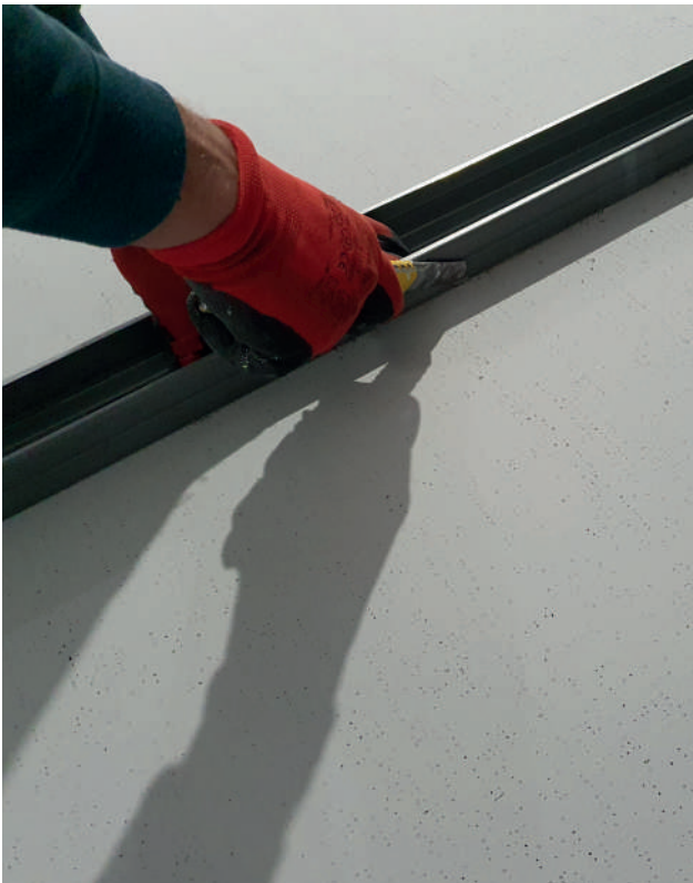
Score and snap method for cutting
