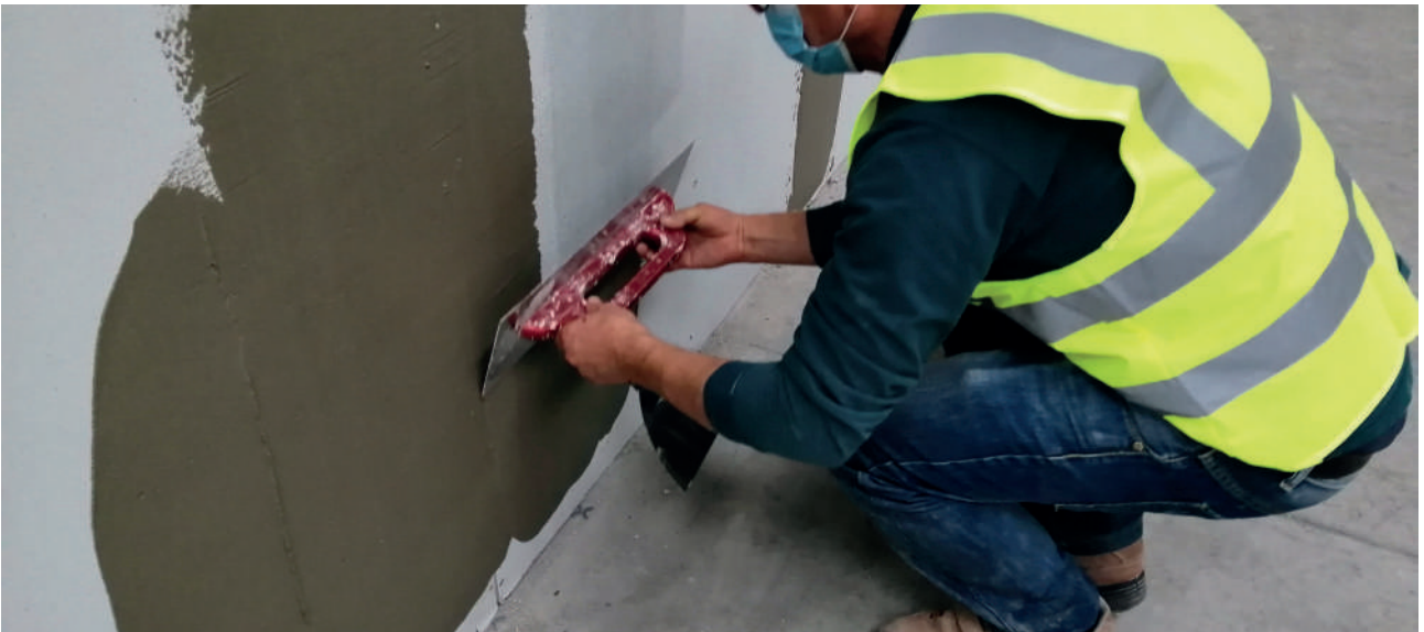
Skim coating SECOLITE® Cement Board
