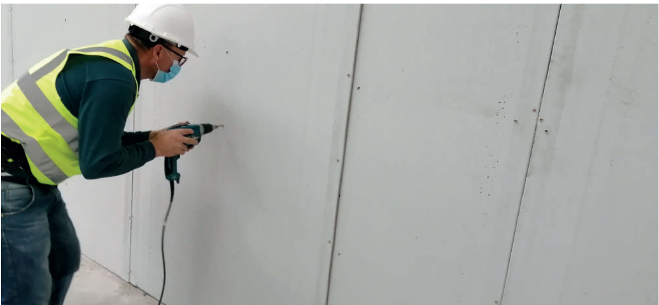
Multilayer vertical installation of SECOLITE® Cement Board
