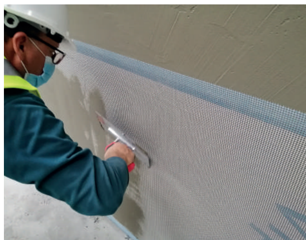
Installation of SECOLITE® Reinforcement Mesh
