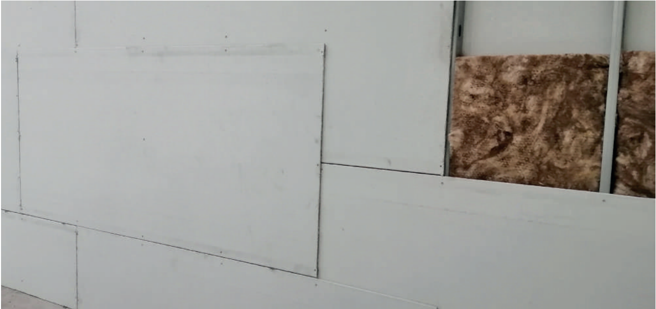
Multilayer horizontal installation of SECOLITE® Cement Board
