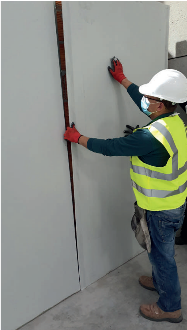
Installing SECOLITE® Cement Board
