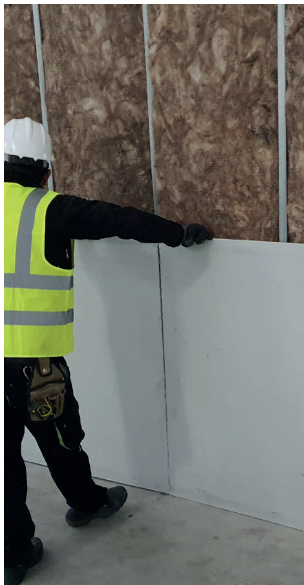
Horizontal installation of SECOLITE® Cement Board
