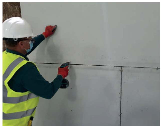
SECOLITE® Cement Board with correct board stagger
