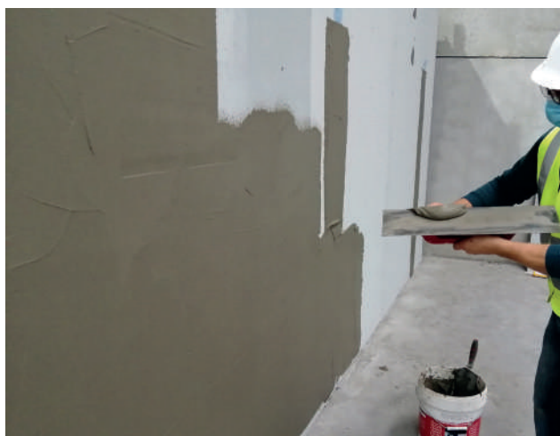
Skim finishing of SECOLITE® Cement Board with SECOLITE® Skim Finish
