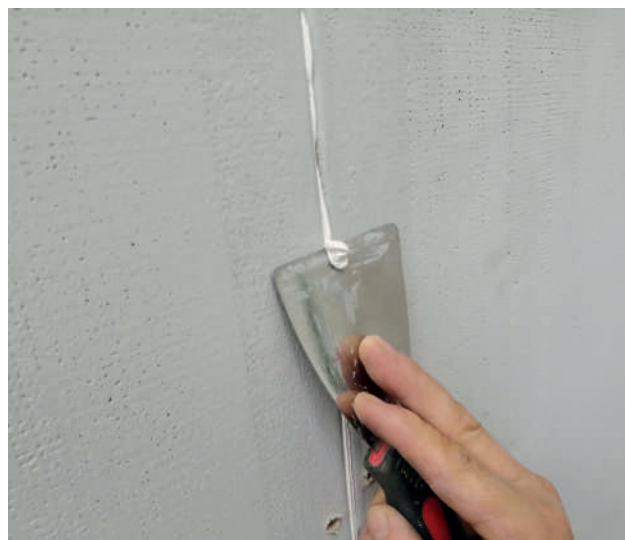
Removing excess SECOLITE® Joint Adhesive
