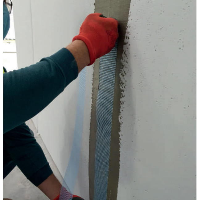
Installing SECOLITE® Joint Tape
