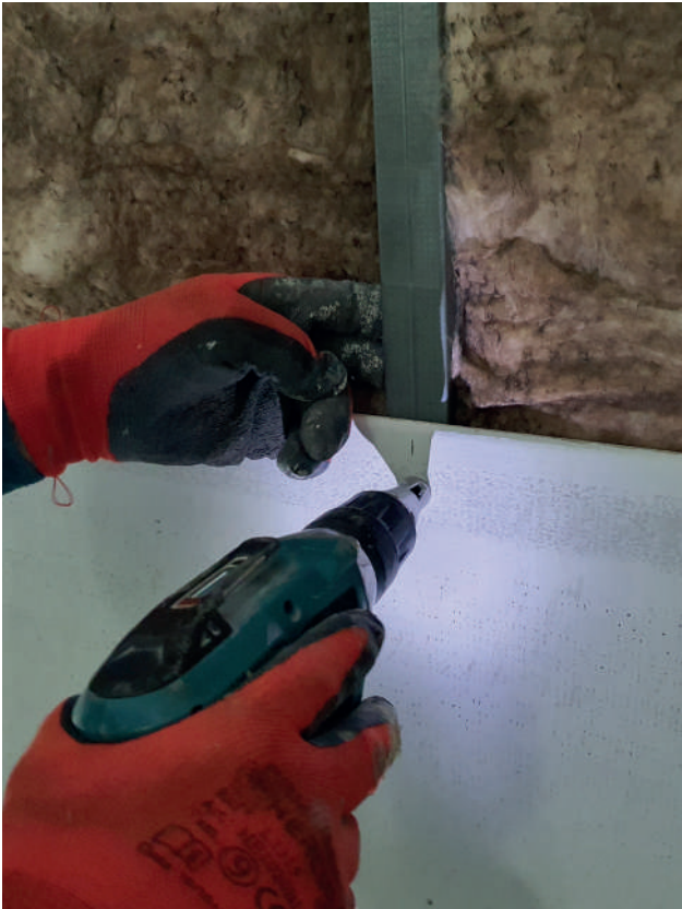
Fastening SECOLITE® Cement Board with SECOLITE® Screws
