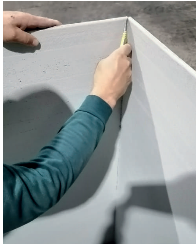
Score and snap method for cutting
